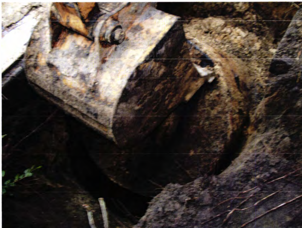
Picture 2: UST 532LaurelBB removal in progress.
